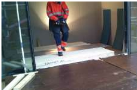
The scaffold needed a stable floor, 1 inch steel was used
