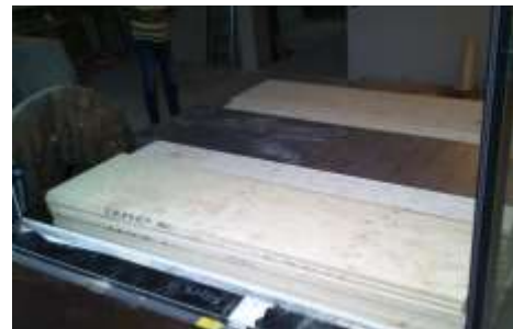
On the inside a floor was built with plywood to make it even against the ledge of the window
